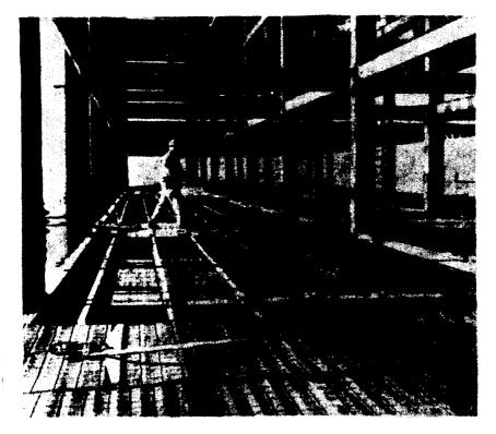
Fig. 28 OPEN WEB FLOOR JOIST INSTALLED AND BRACED
