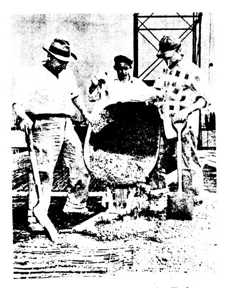
Fig. 31 Placing Concrete Floor Slab Above Open Web Joists (Photograph by courtesy of American Institute of Steel Construction).
