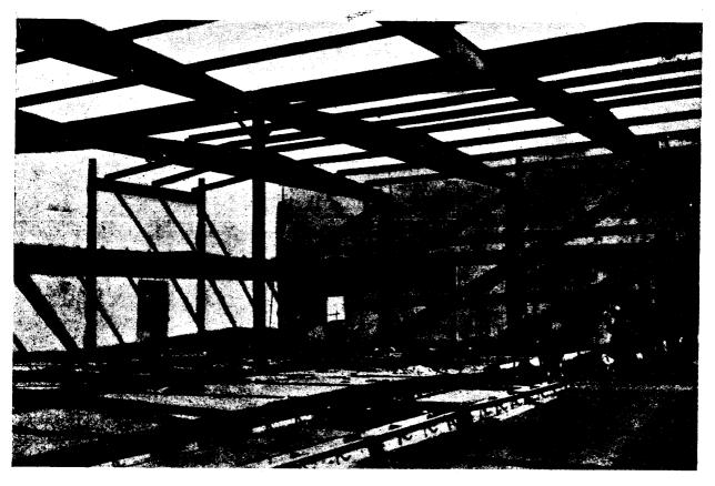
Fig. 34 Tapered Roof Construction (Photograph by courtesy of American Institute of Steel Construction)
